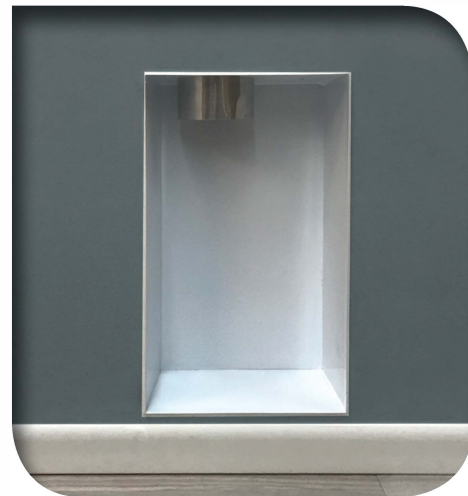
Finish with caulking, no trim ring needed.
